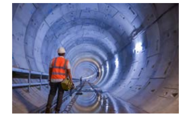
Pressurized water tunnels
