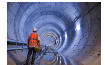
Pressurized water tunnels
