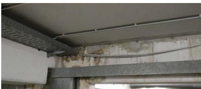
Typical Signs of Damage in a Leaking Expansion Joint
