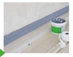
Connection to TPO roofing membranes
