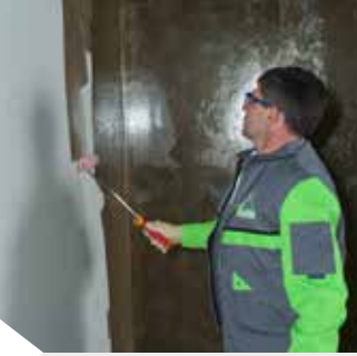
Priming the substrate
