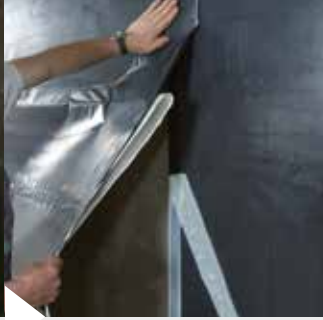
Applying the membrane
