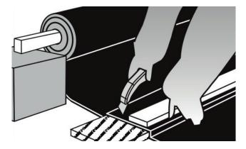
Cut the KÖSTER KSK Membrane using a sharp knife. Cut on top of a wooden board and use a streight edge as cutting support. Wet the blade repeatedly to avoid soiling the blade with bitumen.
