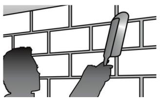
Remove loose particles. The substrate must be clean, sound and solid, free of oil and grease and other substances that may inhibit adhesion.
