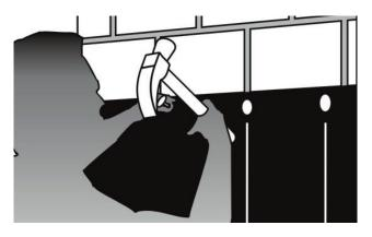
The upper edge of the membrane is fixed in position mechanically. Use large headed nails to fix the membrane in position.
